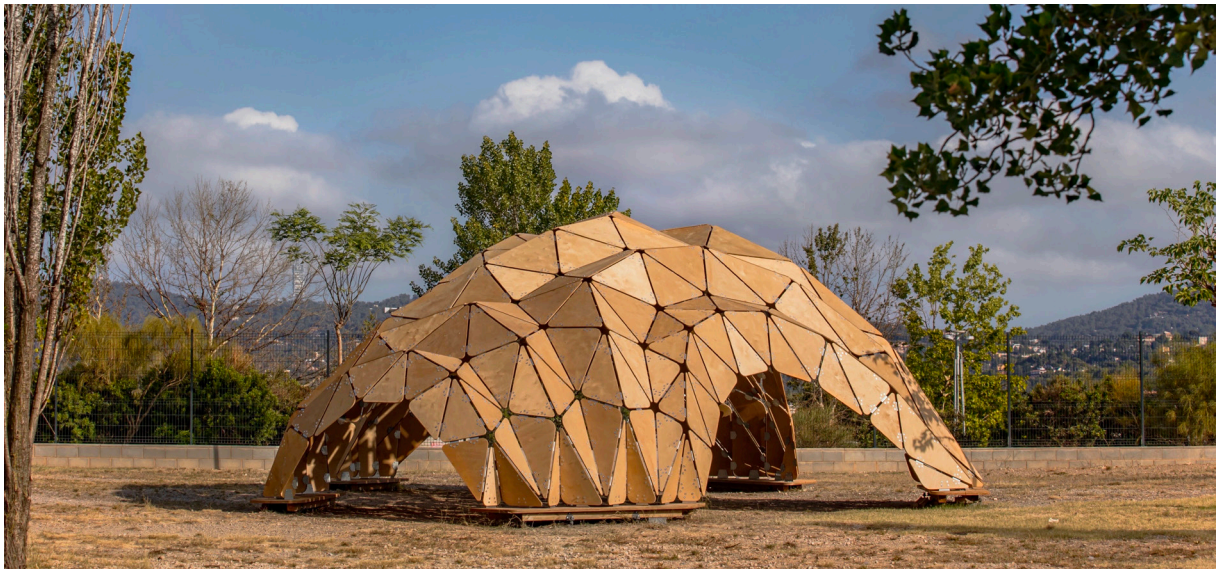
Figure 1: Pentaura pavilion at Escola Turó de Can Mates in Sant Cugat del Vallès, Spain. Photography by Andrés Flajszer.
