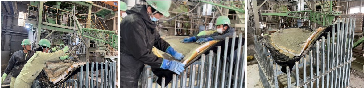
Figure 8: Casting and Compaction of GFRC
